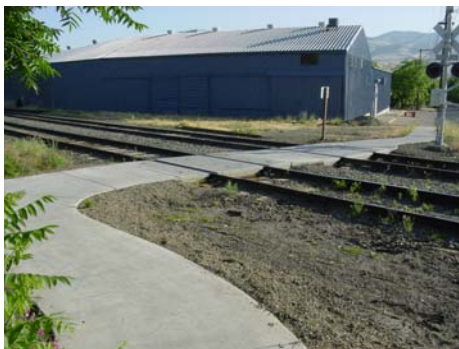
North sidewalk crossing panels
