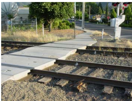
Sidewalk panels being installed on south side of crossing
