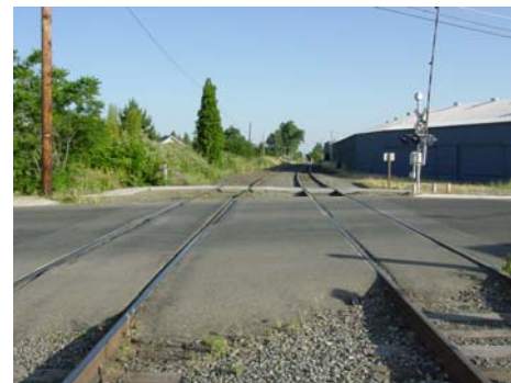
Double track crossing
