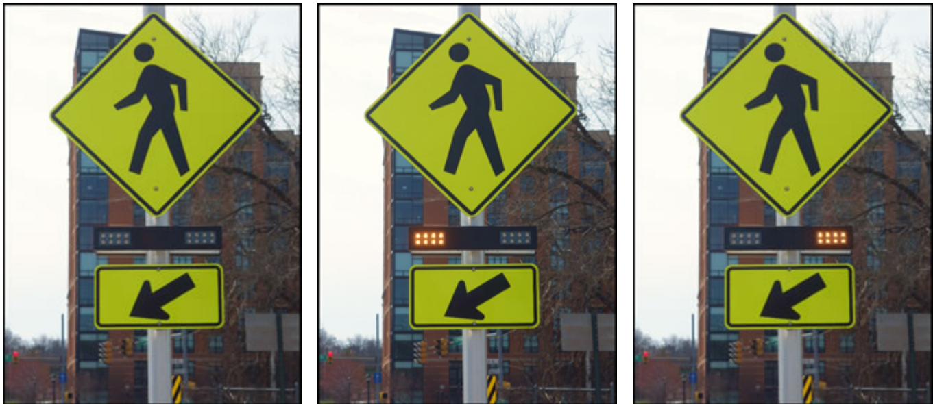
Figure 1. Example of an RRFB dark (left) and illuminated during the flash period (center and right) mounted with W11-2 sign and W16-7P plaque at an uncontrolled marked crosswalk.
