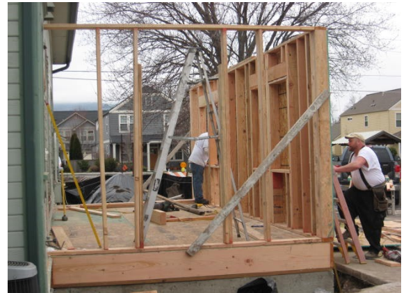
Constructing the Office Addition
