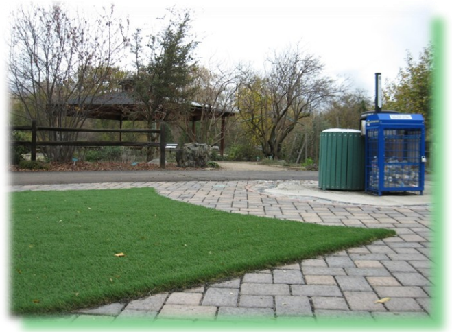
Water Wise Landscaping Demonstration Area Exhibits Artificial Turf and Pervious Pavers
