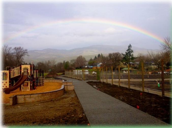
Ashland Creek Park and Gardens Under Construction
