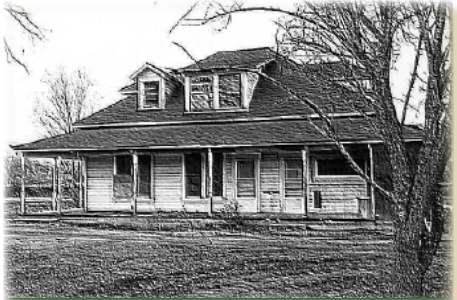
This 1905 farmhouse was renovated and opened as the North Mountain Park Nature Center in 2001.
