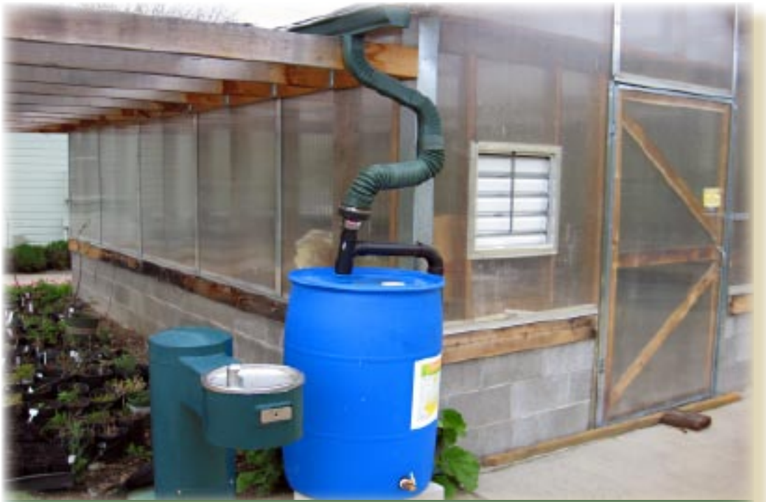
Participants of the fall Rain Barrel Workshop learned how to attach and utilize a rain barrel such as this one attached to the green house at North Mountain Park.
