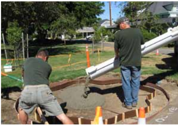
Slab being poured for the recycling area
