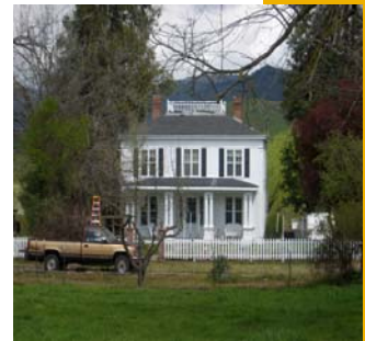
Walker House on E. Main Street.
