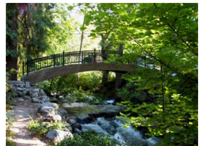
Bridge over Ashland Creek in Lithia Park
