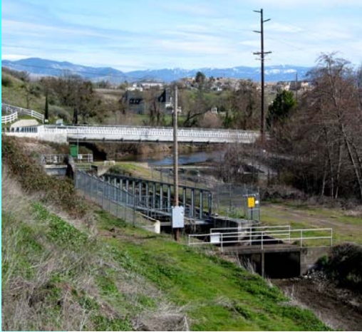
One of three main diversions, TID withdraws water from Bear Creek near Oak Street in Ashland.
