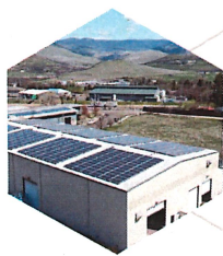
Solar Energy & Photovoltaic
