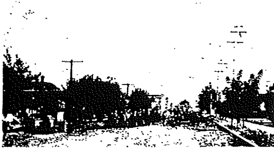
1910 Paving of B Street
