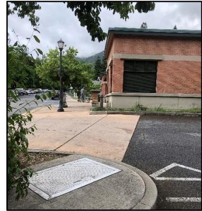
Winburn Lift Station (June 16, 2020)
